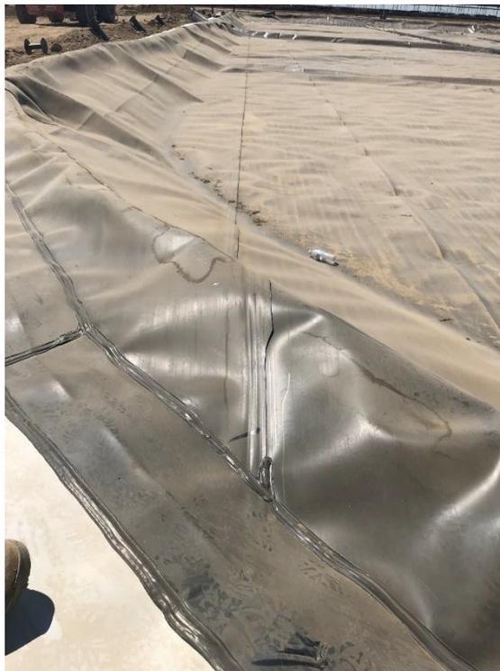
**Image 12.** Details of the digester lagoon cover at K&M Visser Dairy showing welded liners to prevent biogas leakage.
