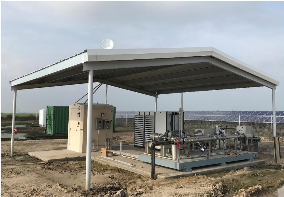
**Image 17.** Biogas conditioning equipment at Little Rock Dairy.
