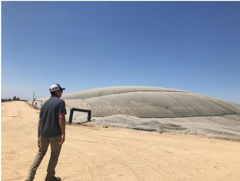
**Image 14.** Covered lagoon digester filled with biogas at the Vander Poel Dairy.
