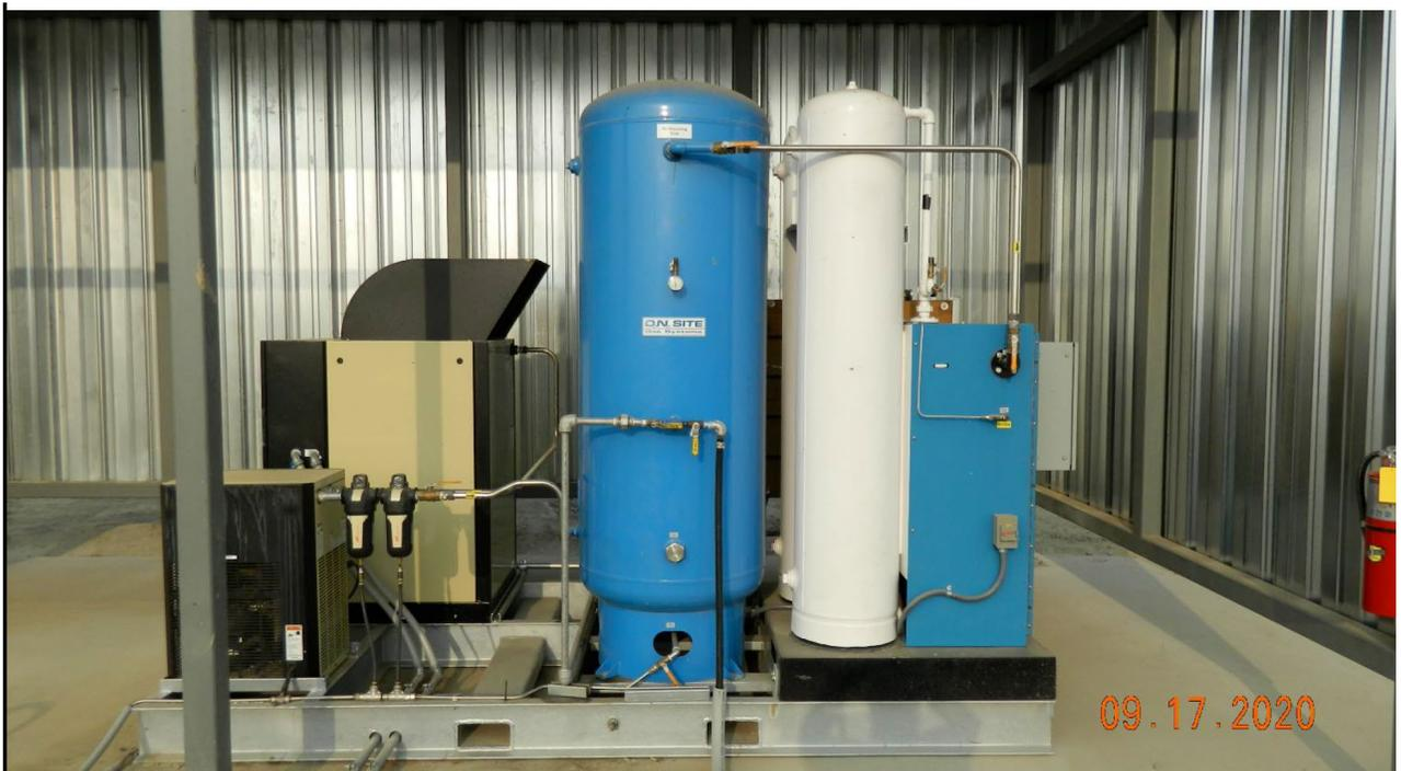
**Image 19.** An oxygen generator skid for biological control of hydrogen sulfide (H<sub>2</sub>S) at Trilogy Dairy.
