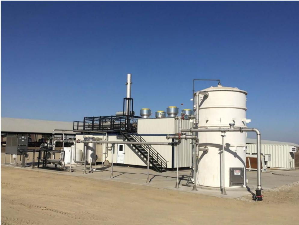
**Image 7.** Electric generation equipment at the Carlos Echeverria & Sons Dairy Biogas Project.
